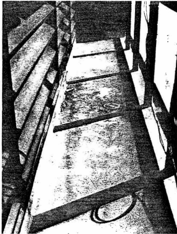
Photo 4.2.5-8 Handrail Post - Exterior Walkway at Junction Level
